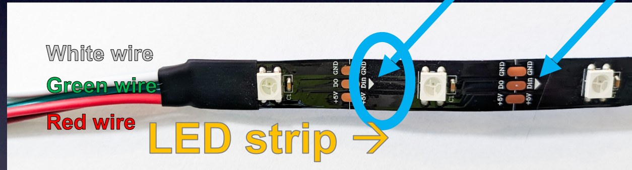
The Input side of the LED Strip
